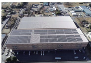
Higashimatsuyama Distribution Center (Saitama Prefecture) On-site PPA Initiatives *PPA: Power Purchase Agreement
