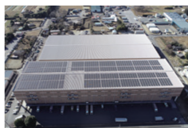
Higashimatsuyama Distribution Center (Saitama Prefecture) On-site PPA Initiatives *PPA: Power Purchase Agreement
